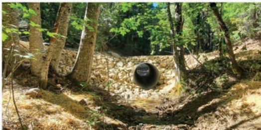
Stream crossing upgrade Before (top) and after (bottom)
