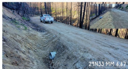
Culvert replacement after fire
