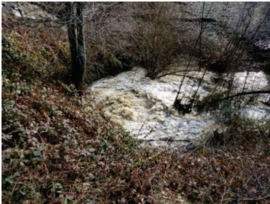
The Yurok Tribe has been awarded funding to design and work through compliance for replacement of the Sky Ranch Road culvert on Oregon Gulch. (Elliot Sarnacki, Reclamation)
