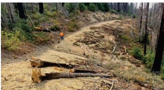
After construction on 30N16B. (Trinity County RCD)
